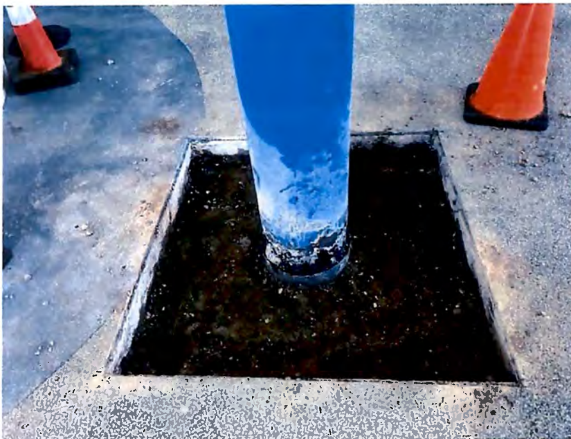
Column-2 excavation. Concrete pier is missing. Three water supply pipes are in the way and must be re-routed around the new concrete pier. This column bears 8'-0" below the floor.
