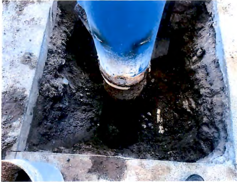
Column-2 excavation. Concrete pier is missing. Three water supply pipes are in the way and must be re-routed around the new concrete pier. This column bears 8'-0" below the floor.
